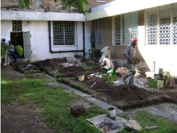
Illustration 17: building in progress
