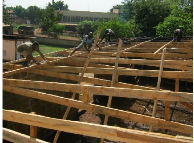
Illustration 19: building of storage
